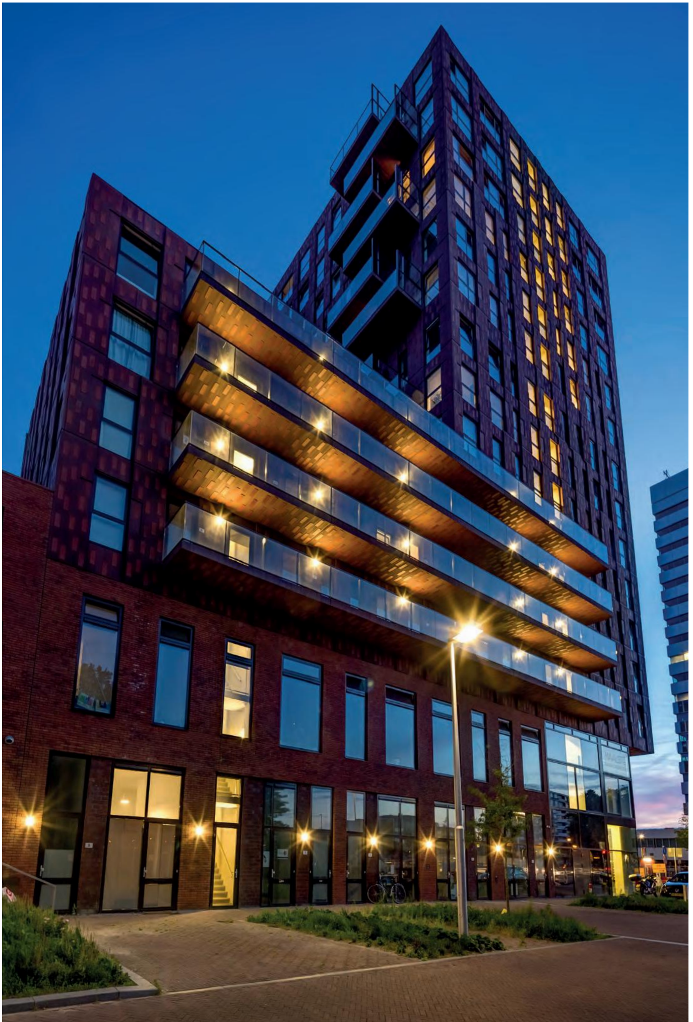
Residential Tower De Verkenner - Utrecht - Netherlands
