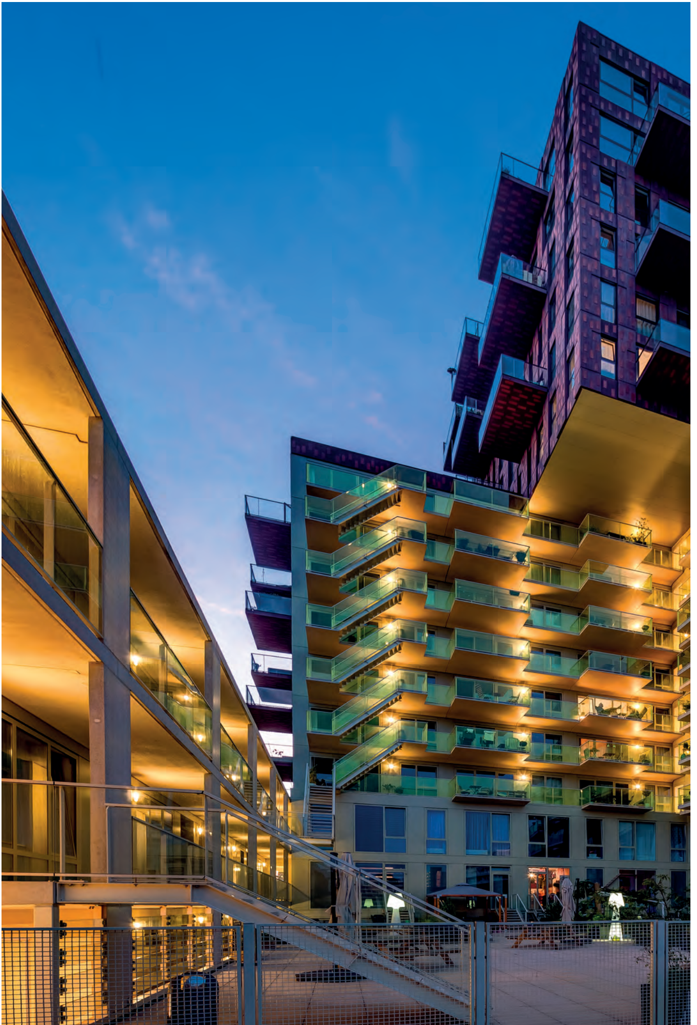
Residential Tower De Verkenner - Utrecht - Netherlands
