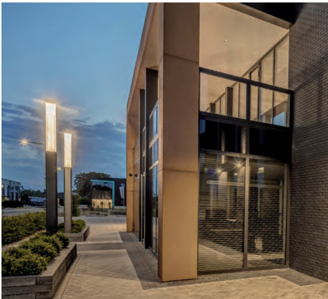
Robri - Wekerom - Netherlands
