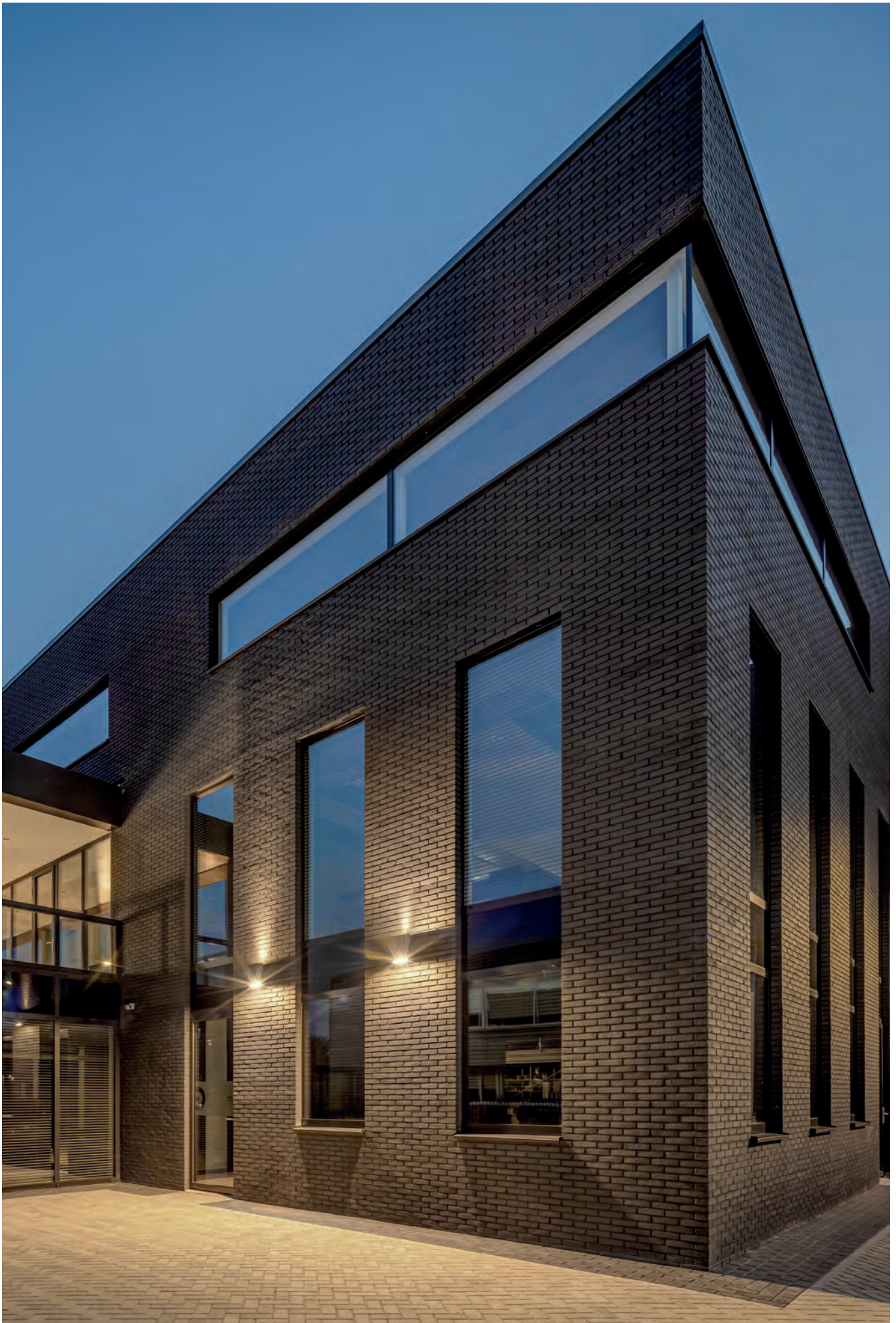
New Building Electrical Wholesaler Robri - Wekerom - Netherlands
