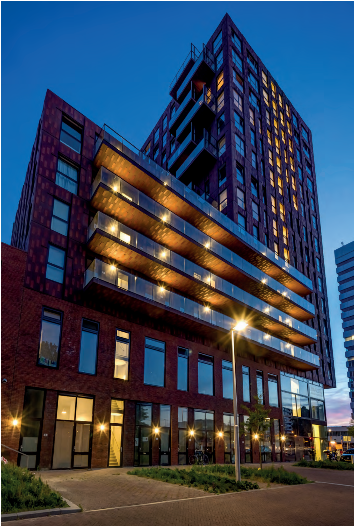
Residential Tower De Verkenner - Utrecht - Netherlands
