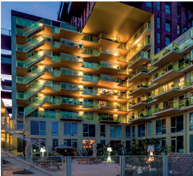
Residential Tower De Verkenner - Utrecht - Netherlands
