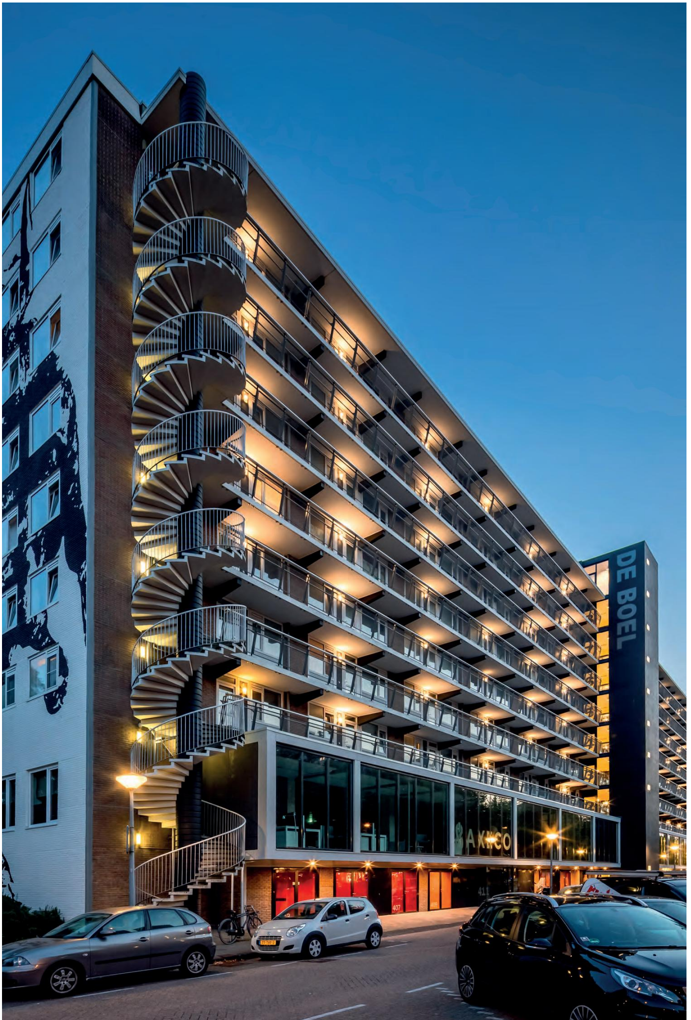
Apartment building De Boel - Amsterdam - Netherlands
