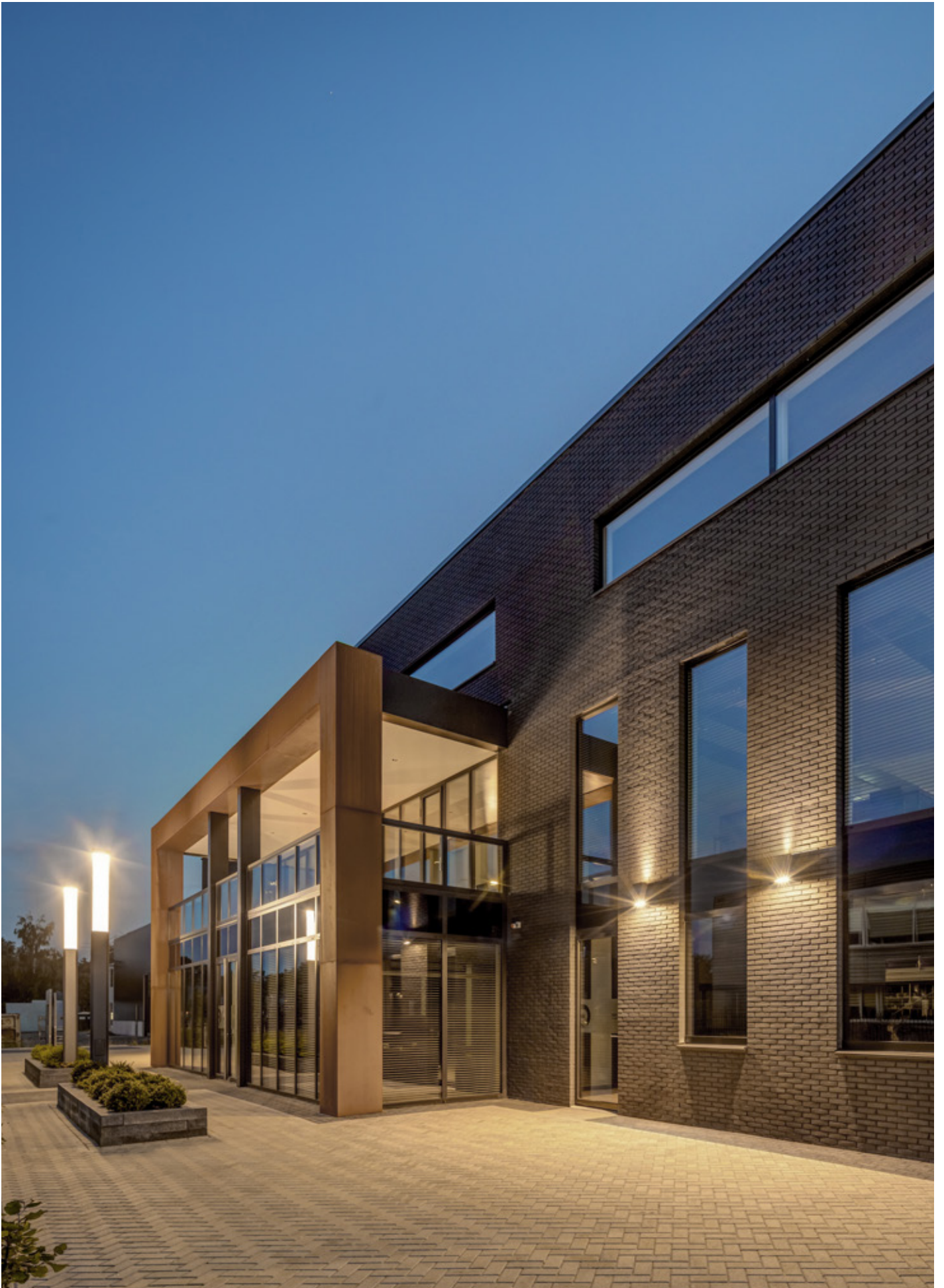
New building electrical wholesaler Robri | Wekerom | Netherlands
