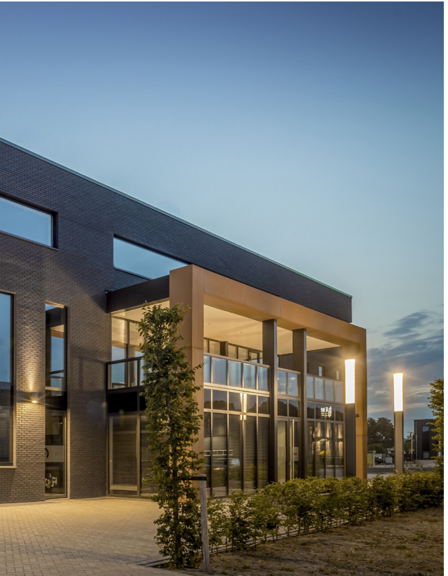
New building electrical wholesaler Robri | Wekerom | Netherlands
