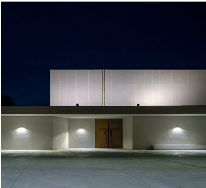
Parish complex - Varignano - Viareggio - Italy
