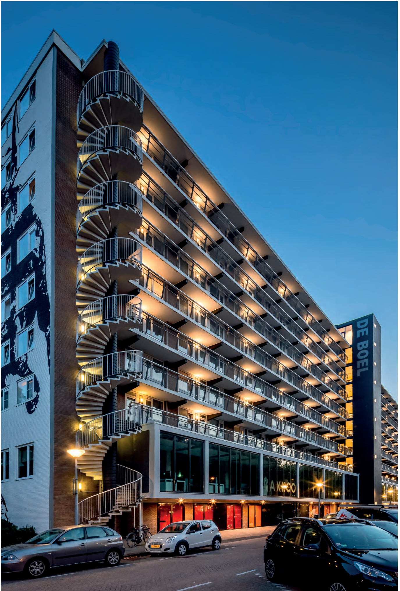
Apartment building De Boel - Amsterdam - Netherlands
