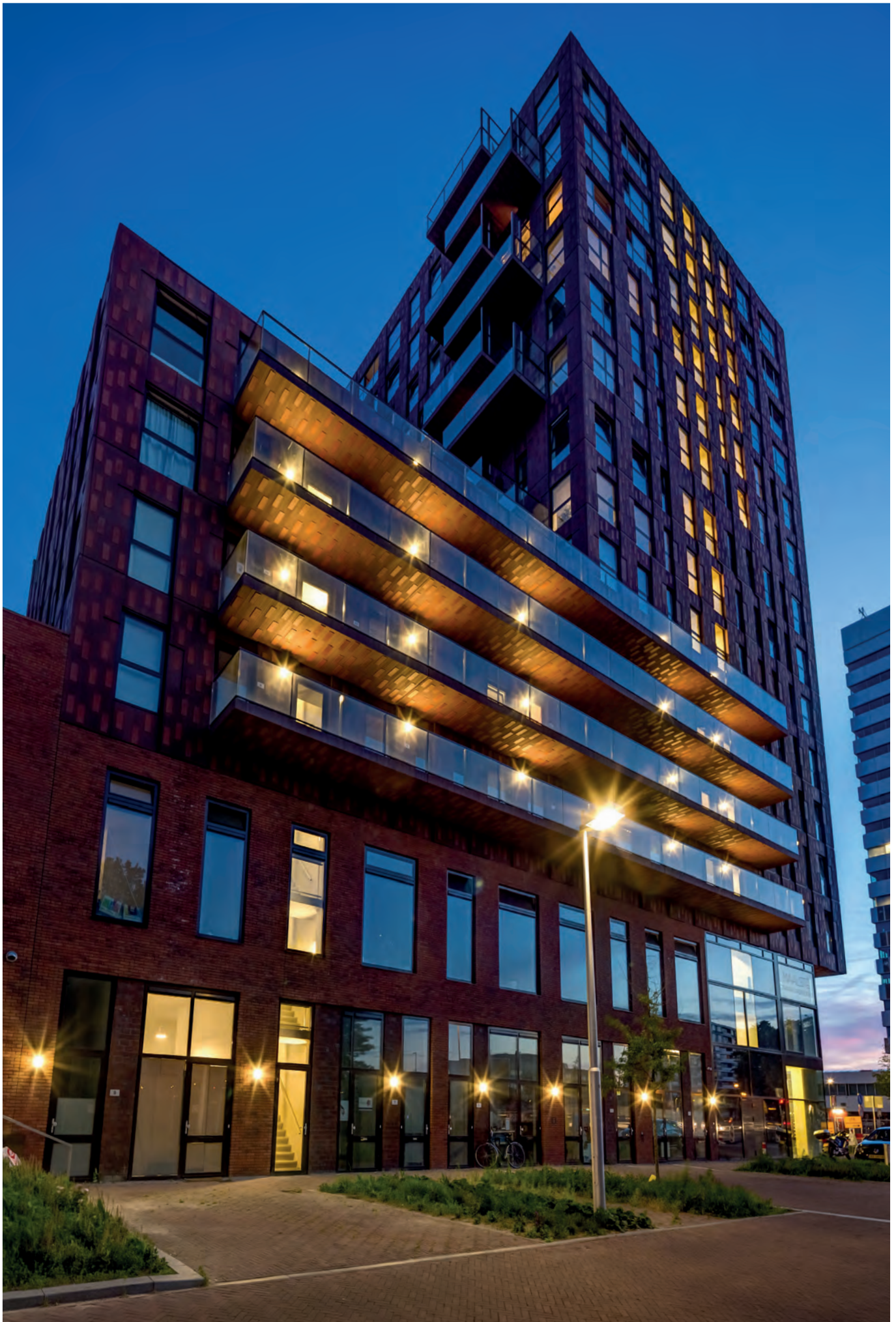
Residential Tower De Verkenner - Utrecht - Netherlands
