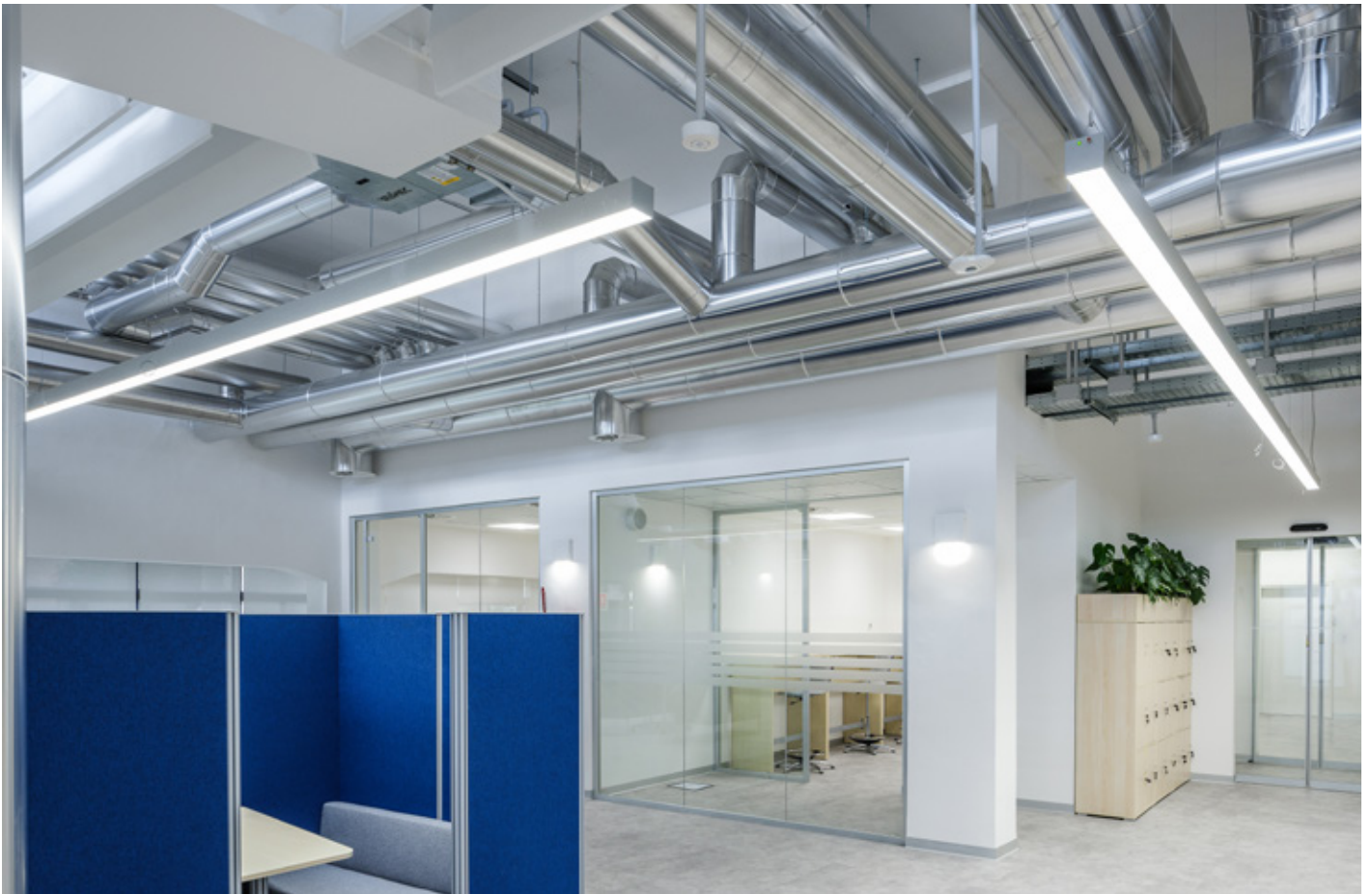
Offices comprensorio Olivetti | Naples | Italy
